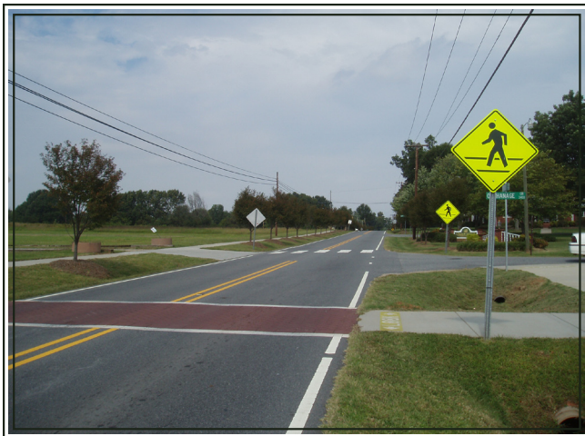
Decorative Crosswalk and Signage on Orphanage Rd.
